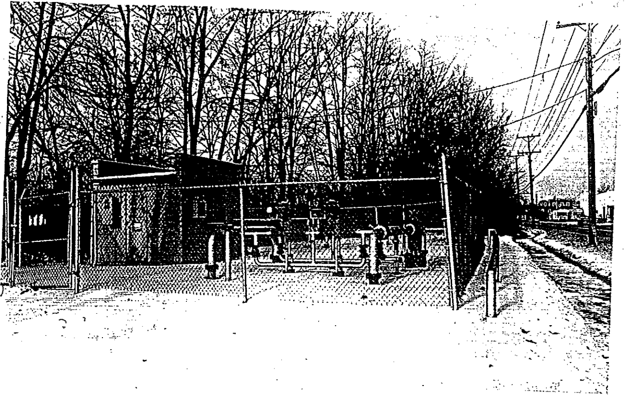
Photograph 55: Gatehouse lot, (37) looking north
