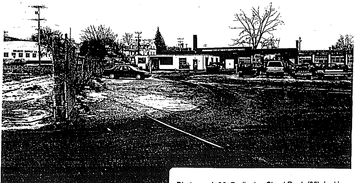
Photograph 38: Burlington Street Dept. (30), looking south; note rail siding in foreground
