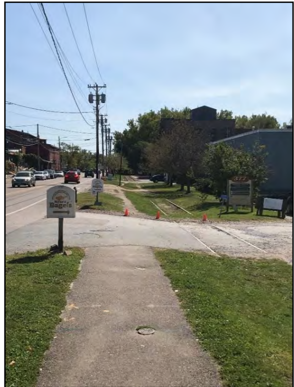
Photo 6-4: Existing Sidewalk Discontinuities
