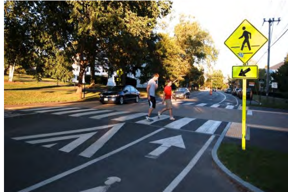
Curb extension, crosswalk and bike racks
